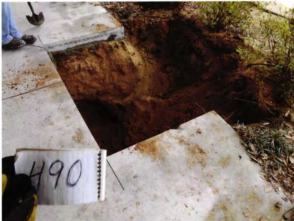
Picture 2: UST 490LaurelBB excavation.
